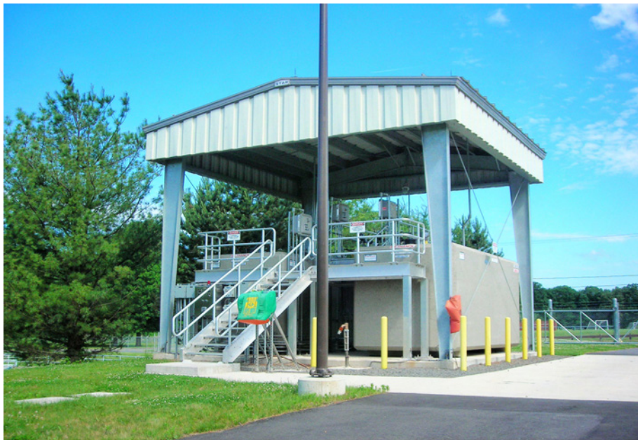
Figure 2 - Cheshire methanol storage and pumping facility
