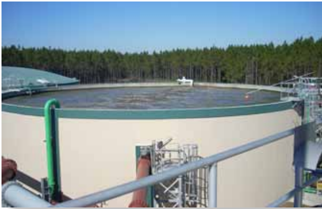
Sequencing Batch Reactor at Blacks Ford WRF, Jacksonville, FL
